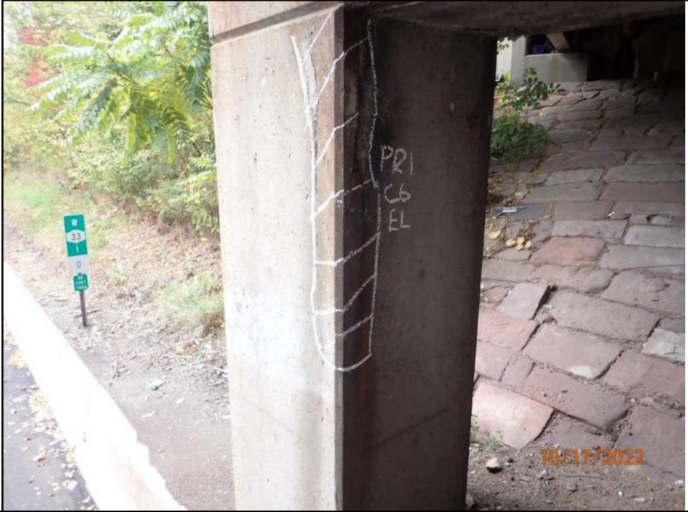
Photo Number: 13 Photo Filename: 13-Vertical cracking in End Left corner of C-6 at
