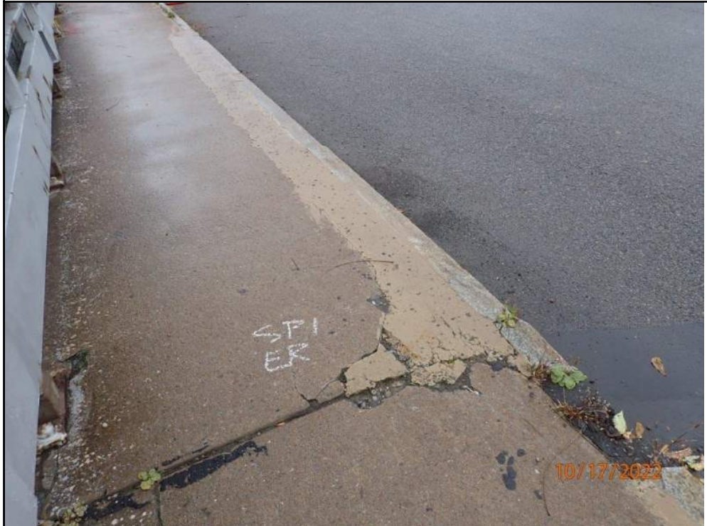
Photo Number: 25 Photo Filename: 25-Typical condition of Joints through
