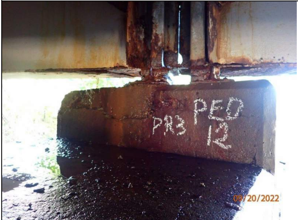
Photo Number: 26 Photo Filename: 26-Active leakage through joint above Bay 11
