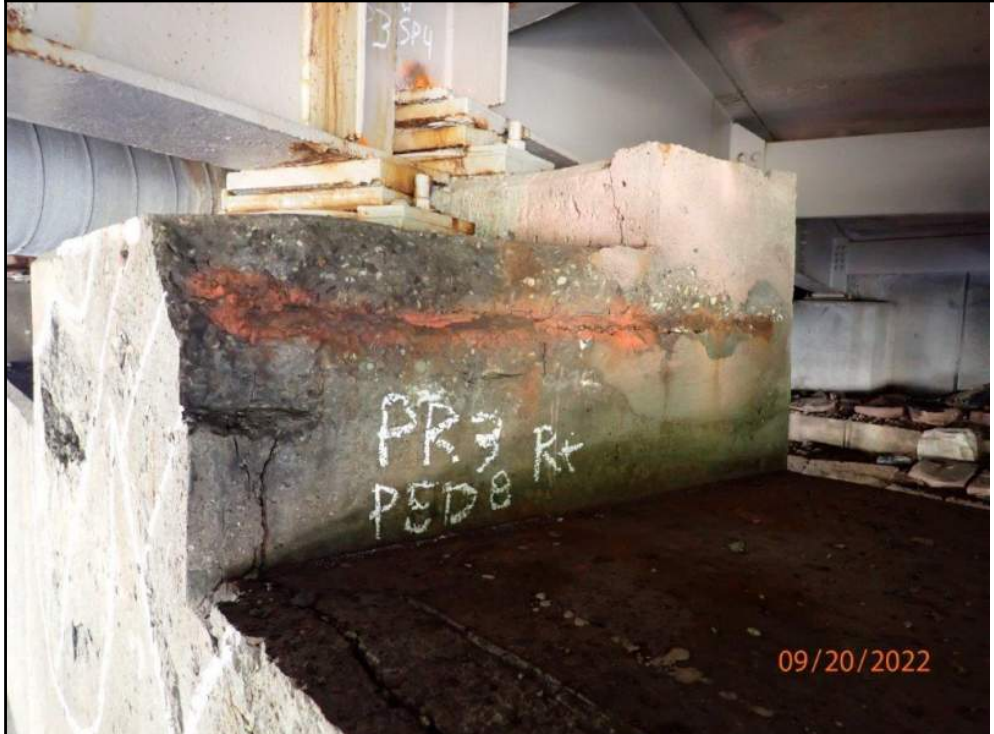
Photo Number: 42 Photo Filename: 42-Right face of G-8 Pedestal at PR-3 spalled
