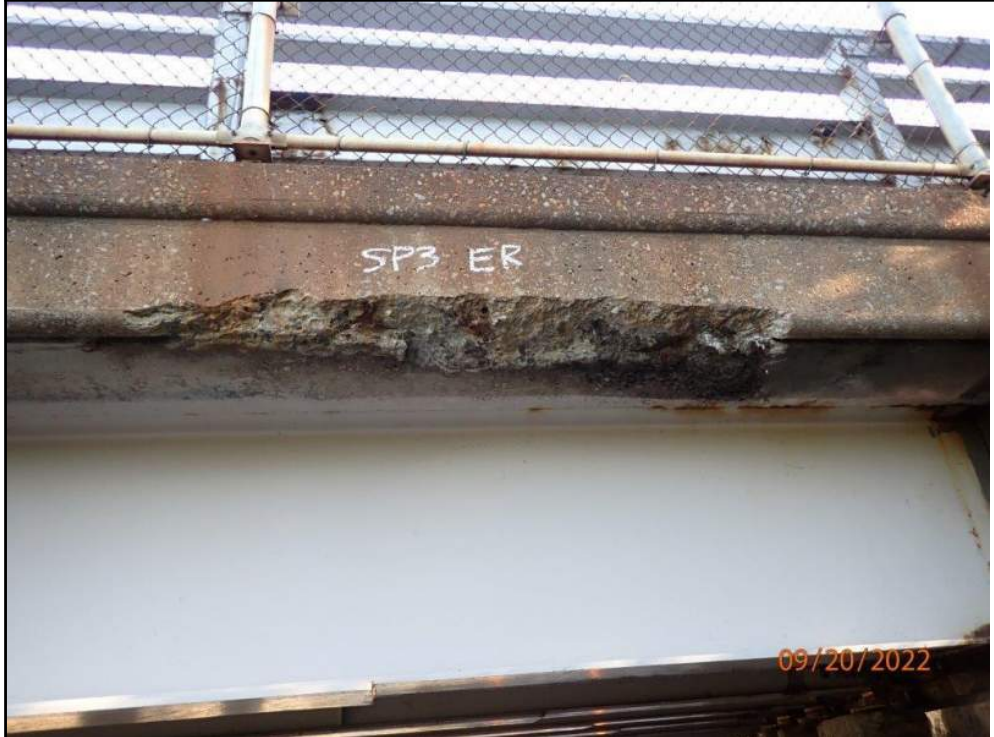
Photo Number: 5 Photo Filename: 5-Bottom corner spall in Right fascia of Span
