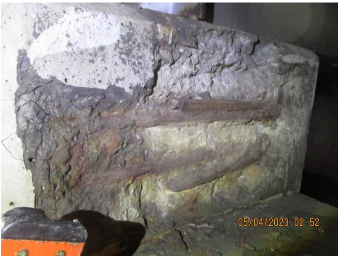
PHOTO 10 LOCATION: PEDESTAL P6 LOOKING SOUTH DESCRIPTION: SPALLS TO CORRODED REBAR ON PEDESTAL
