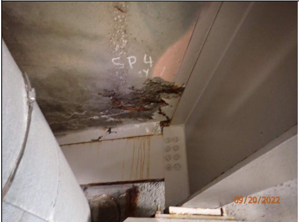
Photo Number: 6 Photo Filename: 6-Spall in underside of Deck in Bay 7 at End
