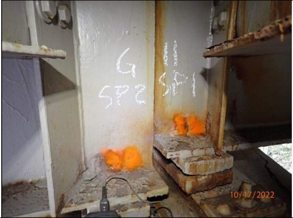
Photo Number: 9 Photo Filename: 9-Painted over pitting in lower webs of G-11
