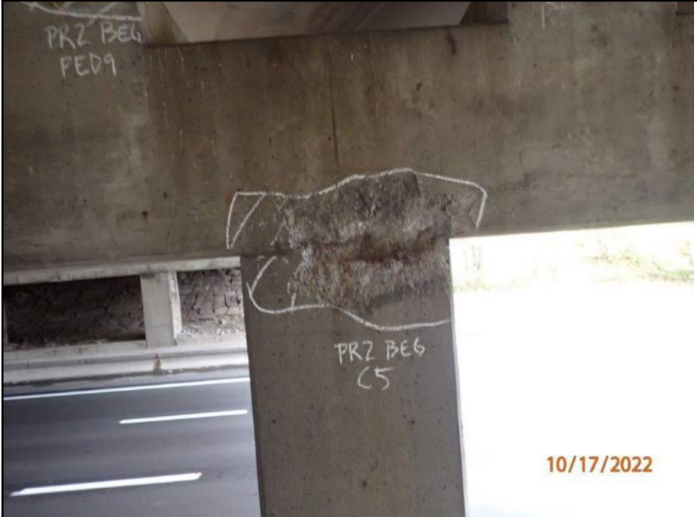
Photo Number: 14 Photo Filename: 14-Spalling near top of Begin face of C-5 at
