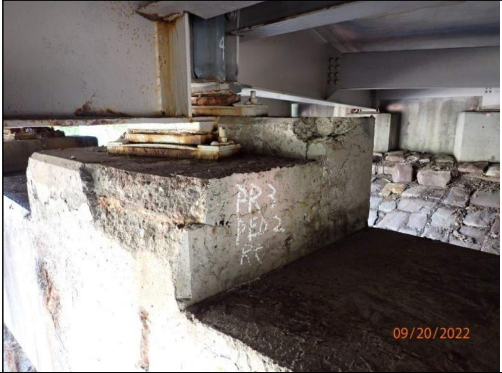
Photo Number: 41 Photo Filename: 41-Begin faces of G-2 Pedestal at PR-3
